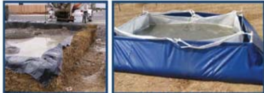
Immovable washout pits
