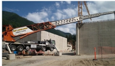
Howard Hanson Dam Seattle, WA
