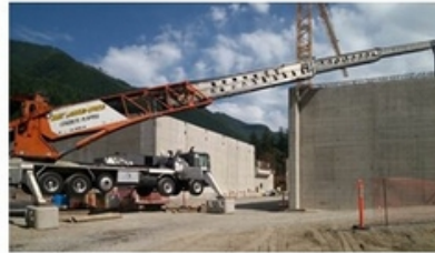
Howard Hanson Dam Seattle, WA
