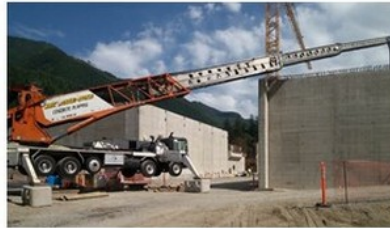
Howard Hanson Dam Seattle, WA
