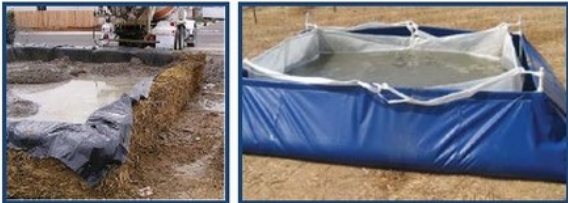
Immovable washout pits
