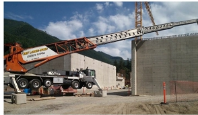
Howard Hanson Dam Seattle, WA
